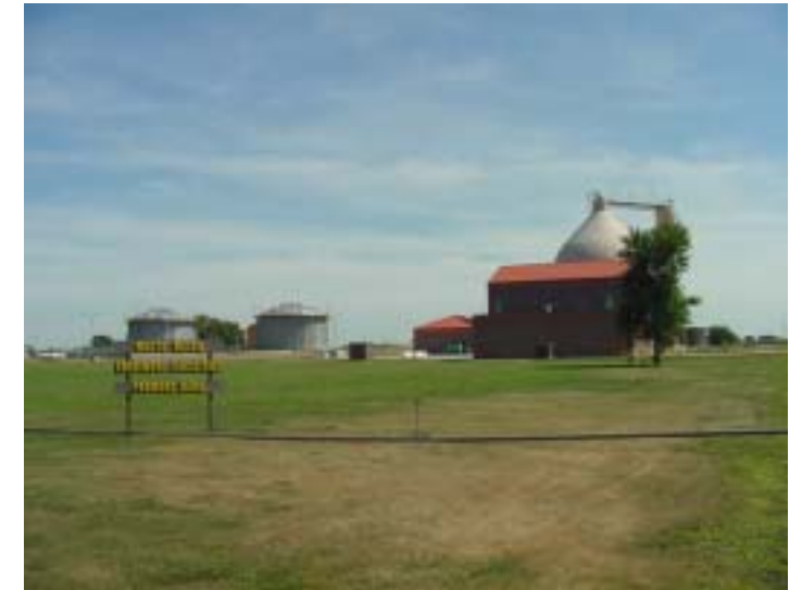
City of Fremont Waste Water Treatment Facility where biosolids are processed.
